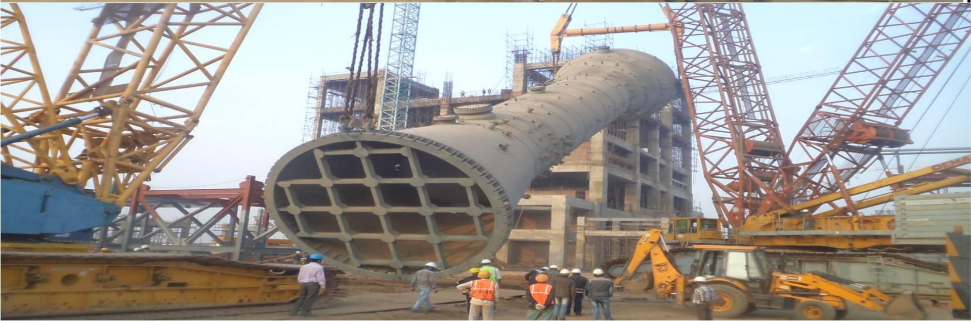
Erection of Polyethylene Reactors at Opal Dahej
